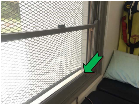
Photo 3. Exterior, first aid room, window frames – non asbestos-containing window caulking.
