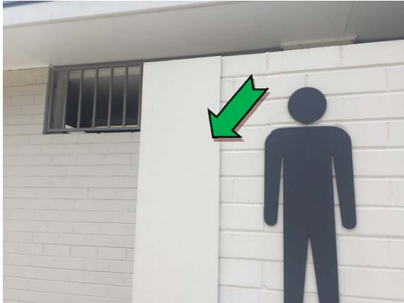
Photo 1. Exterior, toilet block, fascia – non asbestos-containing fibre cement sheeting.
