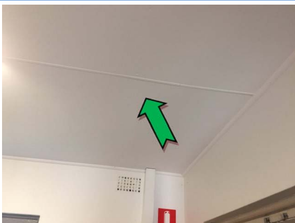
Photo 5. Interior, first aid room, ceiling – non asbestos-containing fibre cement sheeting.
