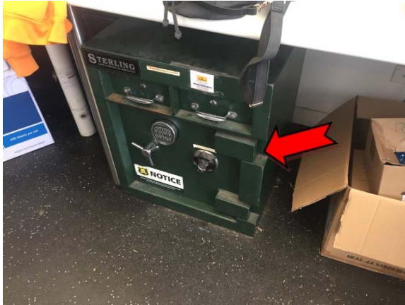
Photo 7. Interior, office, safe – suspected asbestos-containing internal insulation.
